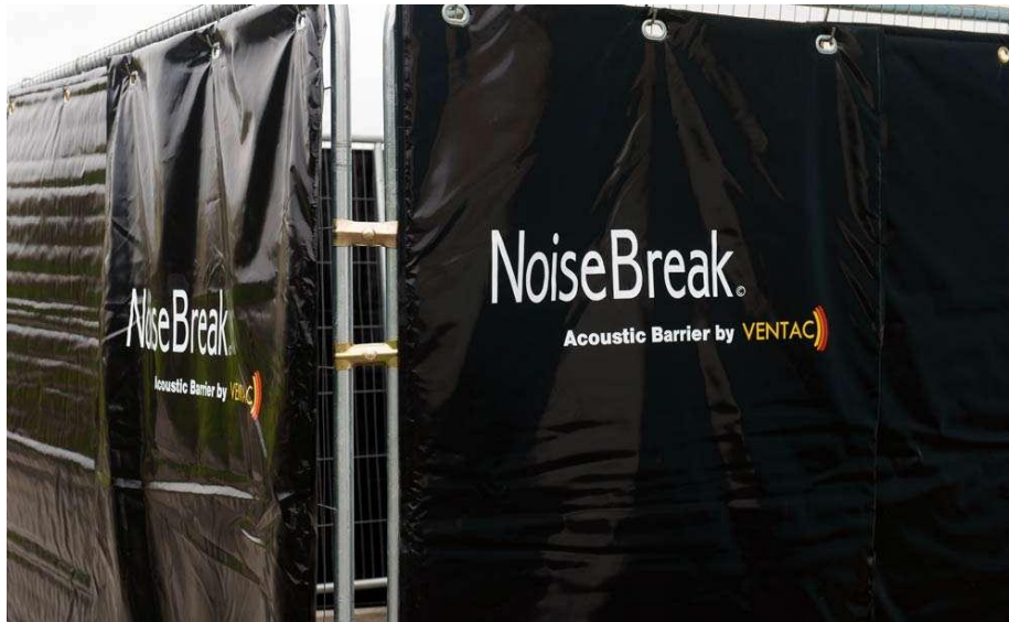
Figure 11.6: Temporary Construction Noise Barrier © Ventac.
